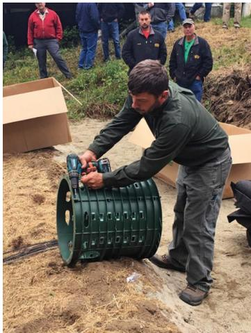
*Mike Carbonneau, owner of Connecticut Valley Design in Littleton, New Hampshire, demonstrates where to screw together the two halves of the EnviroFin distribution unit. (Courtesy of Presby Environmental)*
