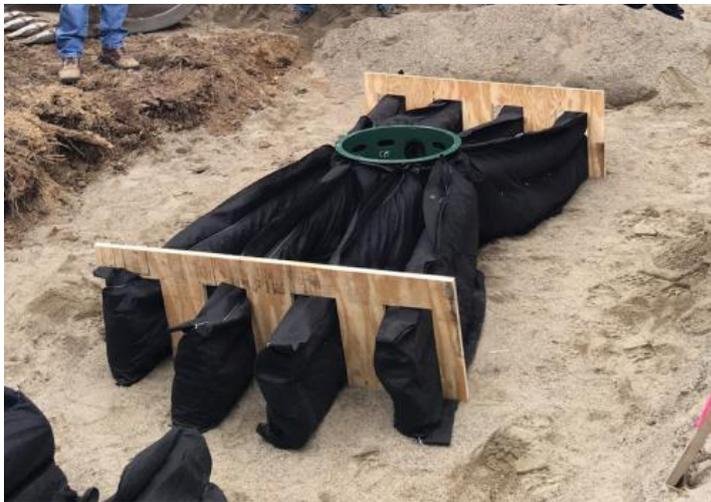
*Two homemade plywood spacers hold the fins in position during backfilling and maintain the required 15cm separation between them. (Courtesy of Connecticut Valley Design)*
