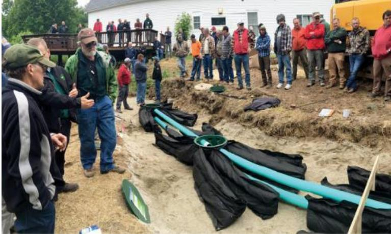
*Some of the 90 attendees observe how multiple Presby EnviroFin distribution units are connected by two 100 mm PVC pipes. The upper one transfers oxygen and the lower pipe distributes effluent. (Courtesy of Presby Environmental)*
