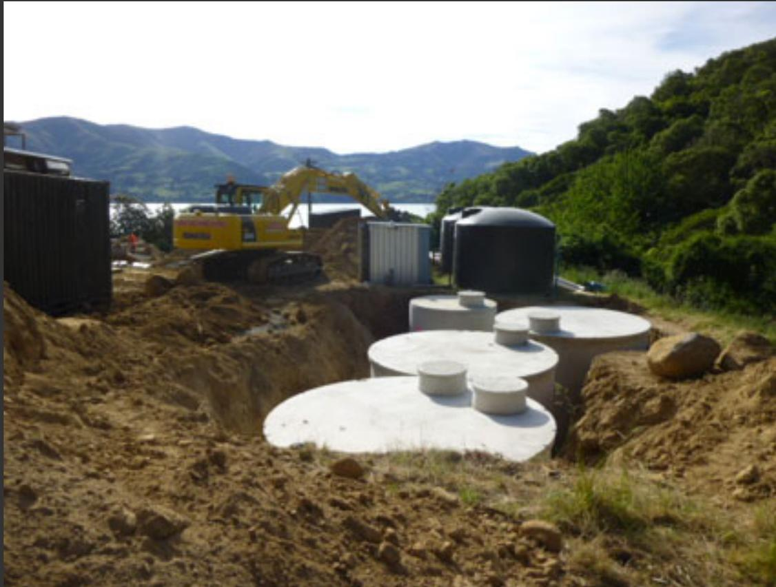
**A string of septic & flow balancing tanks totalling 78,000L.**
