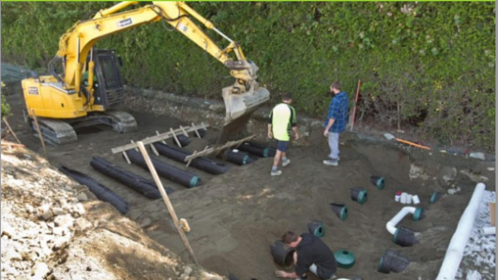
In October this year Greenwood Park Motel and Campground upgraded its wastewater system. Tuffnell Plumbing and Drainage installed an AES system sized to treat 19,000 litres per day. The system was designed by Tasman Consulting Engineers' Ron O'Hara as a replacement for a sand filter system. While AES is often installed to service single dwellings it can be up-scaled to suit. The Greenwood Park installation is the largest AES installation in NZ to date. Full story [here](#)
